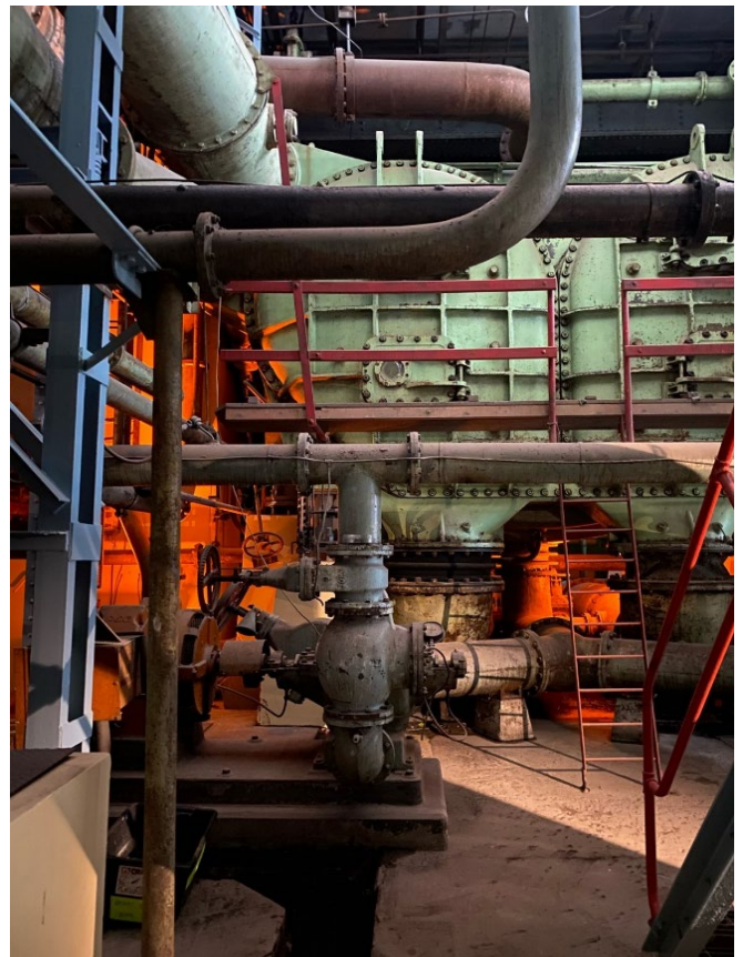
Image Credit: White Bay Power Station, JOC Consulting
