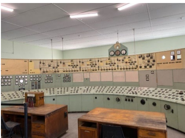
Image Credit: White Bay Power Station, JOC Consulting
